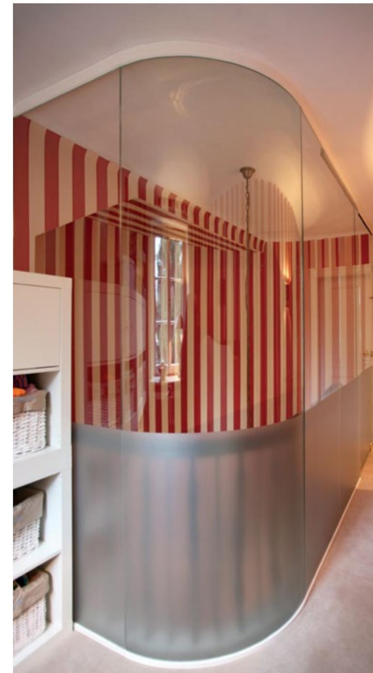
off the stairway area and rule out falls, the Ahrensburger Glasbau company installed a complete wall of safety glass.
